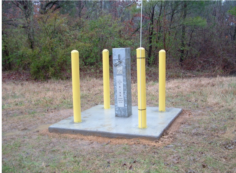
Photo 5 Completed Well B-8R.
