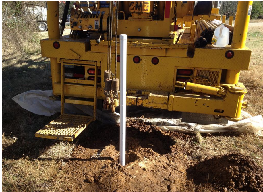
Photo 2 Typical completed well.
