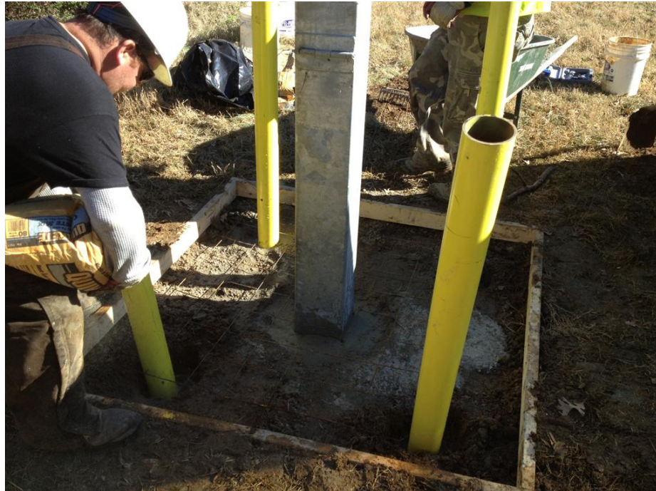
Photo 3 Typical surface protection construction.
