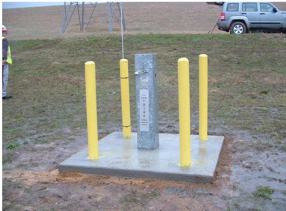
Photo 4 Completed Well B-6R.
